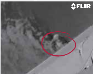
Captured gas leak from production site.
