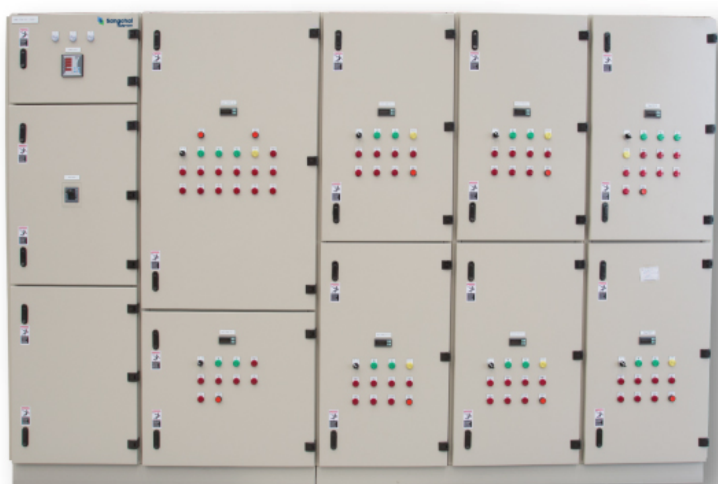
MCC : Motor Control Center
